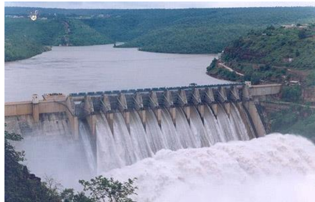
Fig-8(b) Photograph of a hydropower project (CLIMATE HOME NEWS, 2013)
