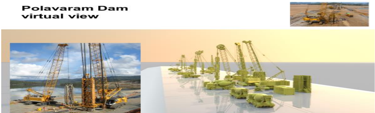
Fig:8-Machinery of Diaphragm Wall and Placement at Dam Site
