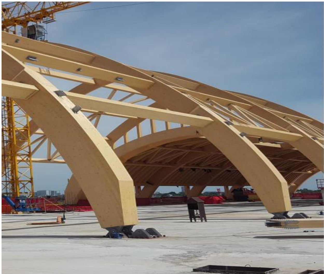
Fig. 2 Anchoring arrangement.
