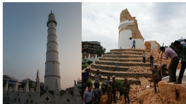
Fig. 7 a & b. Dharahara Tower before & after quake
