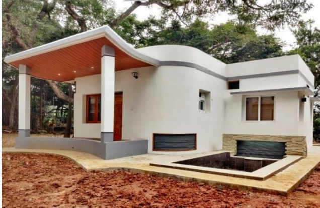
Fig. 2: One story house 3D printed house by Tsvasta [21]
