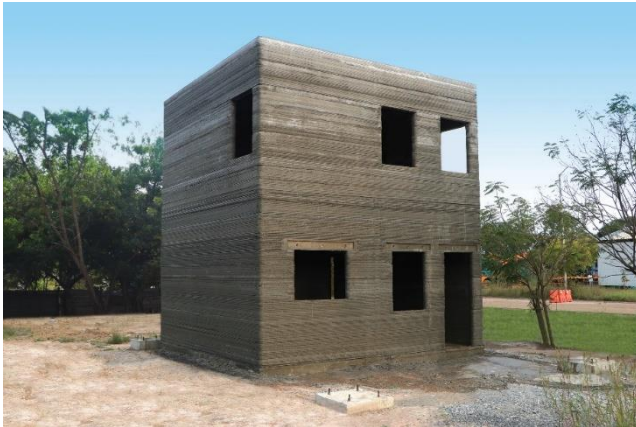
Fig. 3: Two story house 3D printed house by L&T [22]
