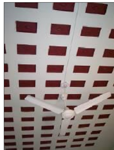
Figure – 5: View of ceiling of RCC Filler Slab
