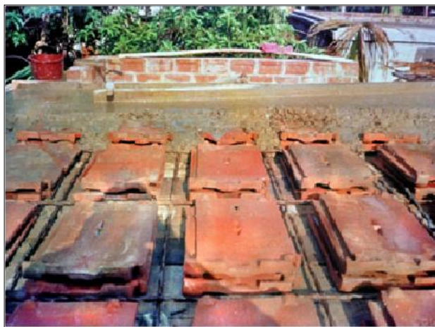
Figure – 4: RCC Filler Slab during casting
