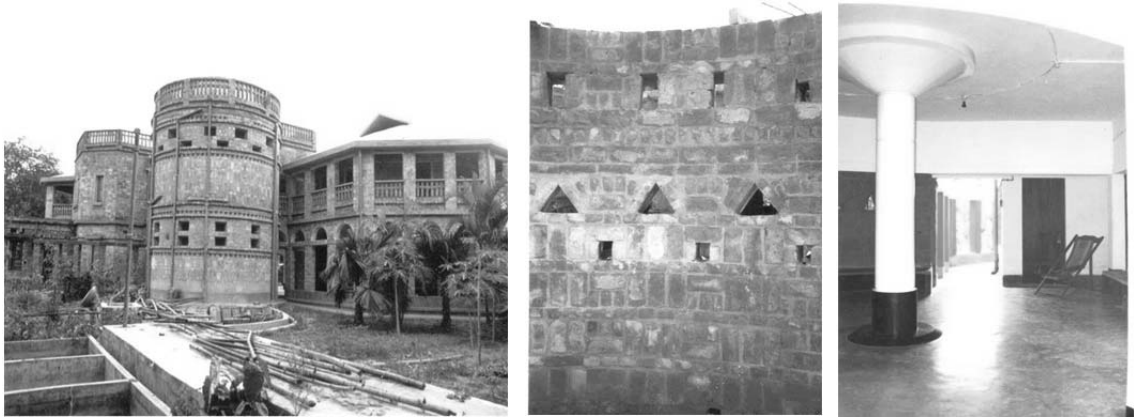
SWANIRVAR TRAINING CENTRE AND OFFICE AT BADURIA
