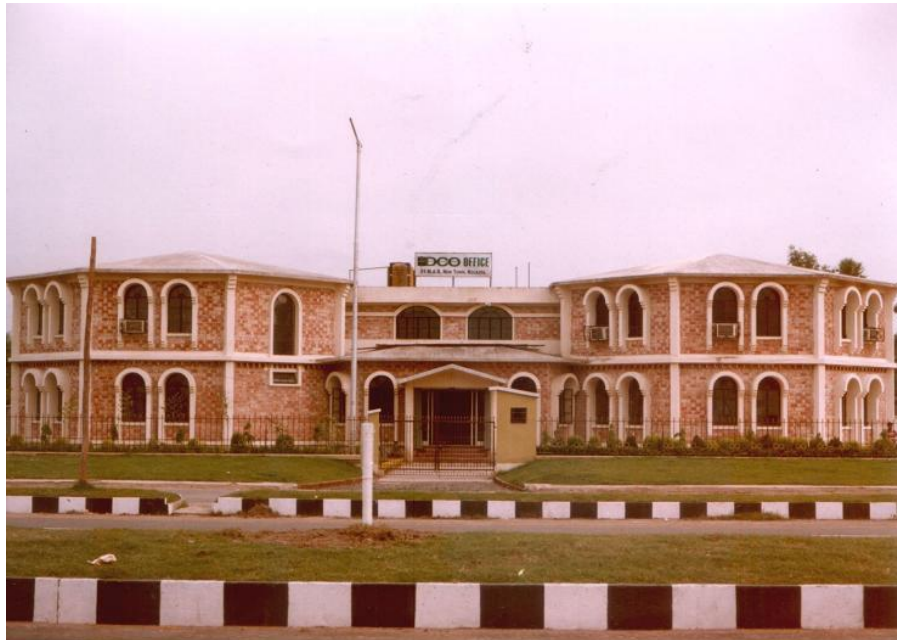
Two-storied Office Building with Rat-trap bond wall
