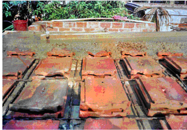
Filler Slab Roof under construction
