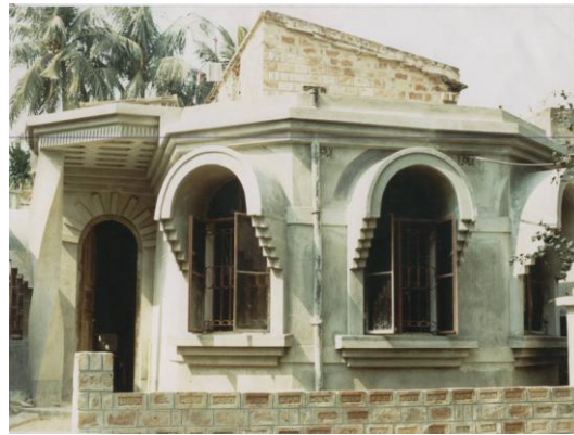
Brick Corbelling Picture – 5 (Source: FOSET)
