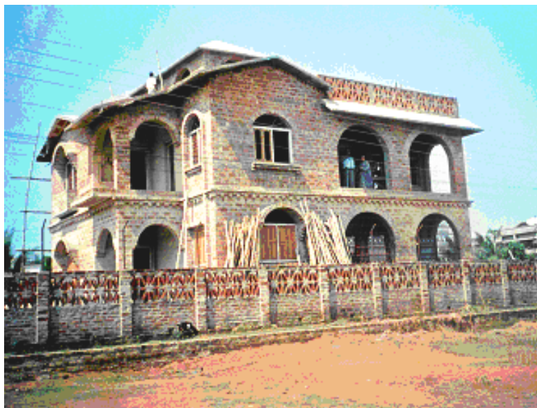
Two-storied Residential Building with Rat-trap bond wall under construction
